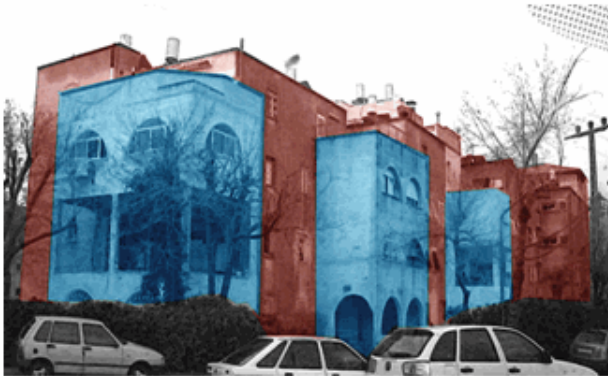
Figure 5 – Apartment extensions without supervision and not in accordance with the plan regulations that apply in the area.
