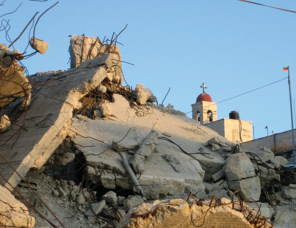
The rubble of a Beit Hanina home after its owner demolished it due to Israeli pressure. ©PCC
